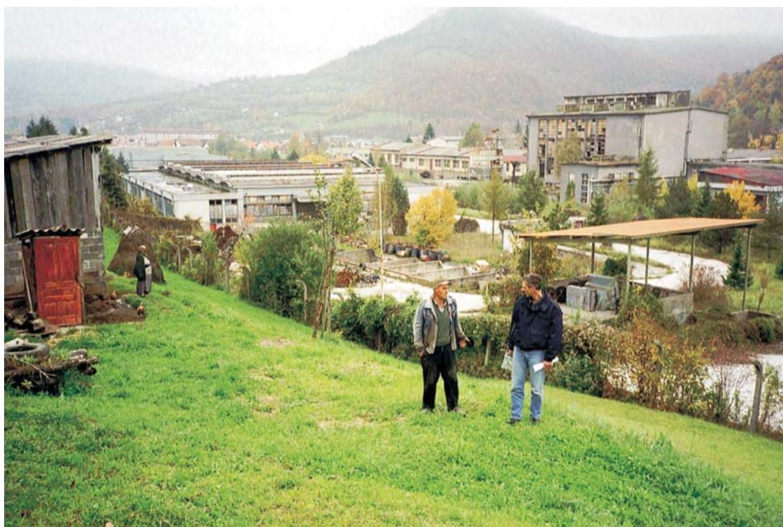
An overview of the Hadzici Tank Repair Facility from a neighbouring home
